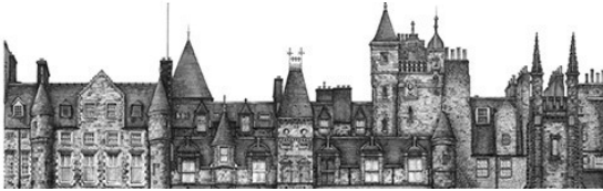
002 Rooftops of the Mound
